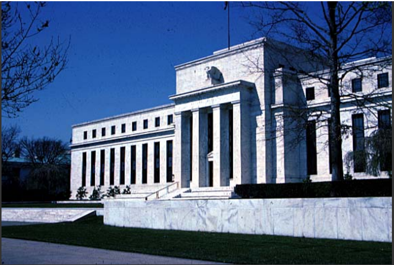
The Federal Reserve Building in Washington DC
